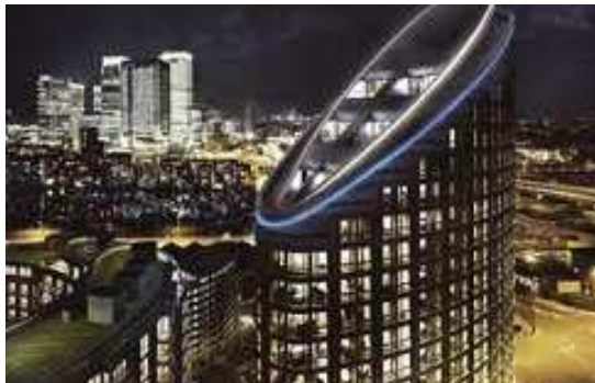
Ontario Tower - London
