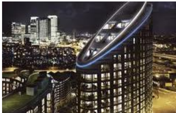
Ontario Tower - London
